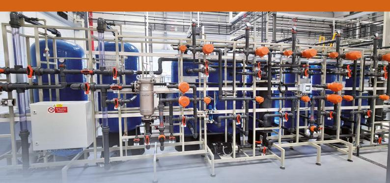
Ion-exchange Circulation Stations (ICS) for the treatment and recycling of rinse water. In a closed circuit, used rinse water is continuously purified (demineralized) and returned to the production process.
